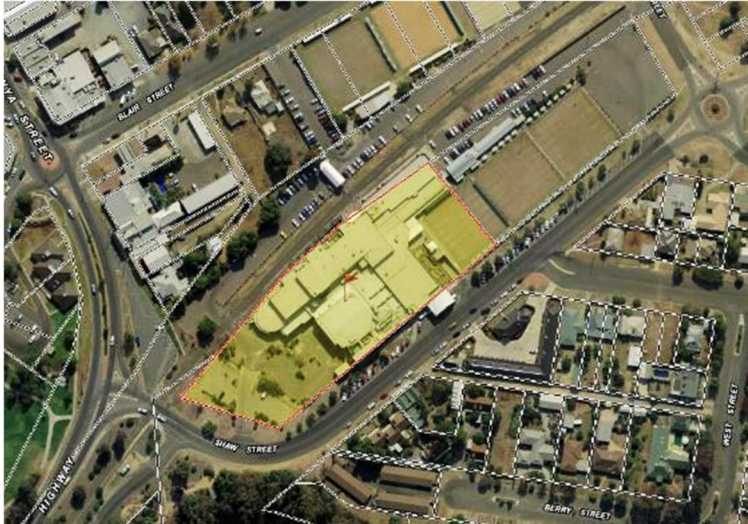
Figure 6 Aerial of the subject site (outlined in red and shaded yellow) containing the main Moama Bowling Club building and carpark showing the bowling greens located to the east (Source: SIXViewer)
