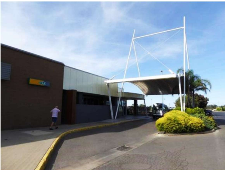
Figure 11 View of the entrance from Shaw Street
